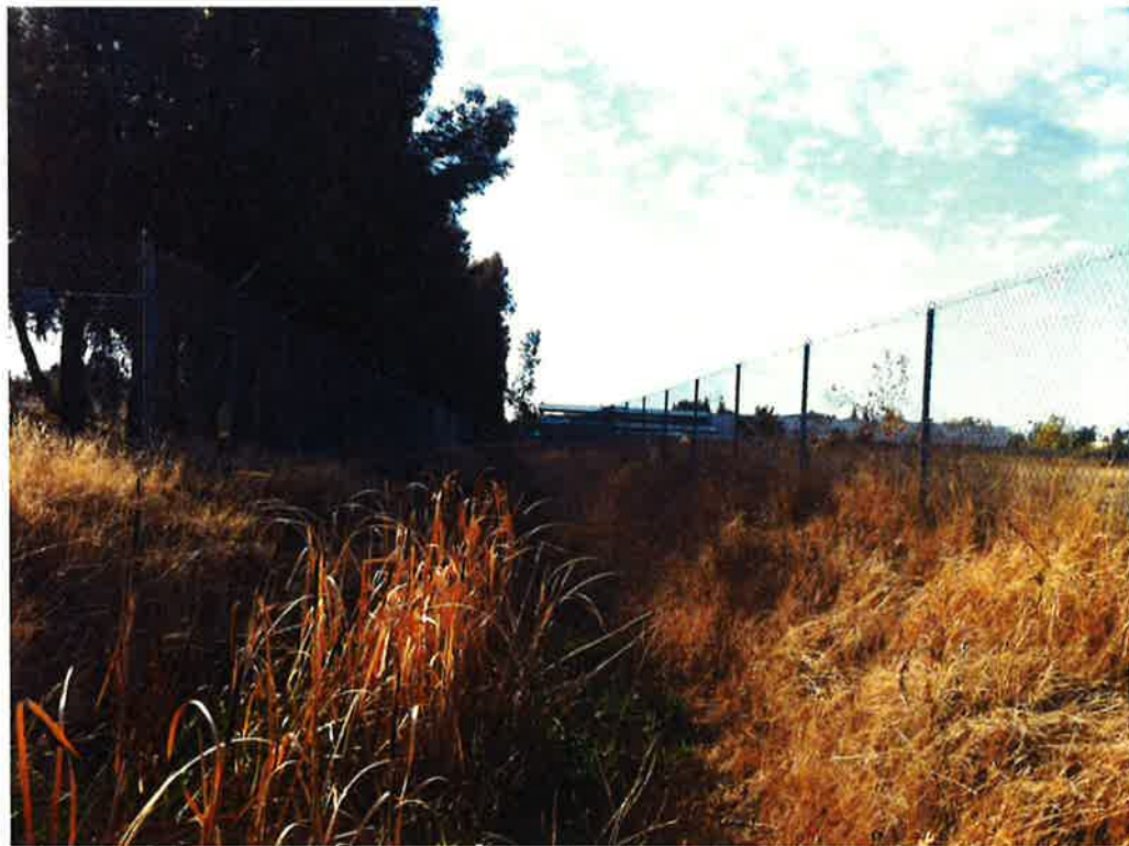
View facing south at the portion of the Site that appears to consist of the unlined drainage swale.
